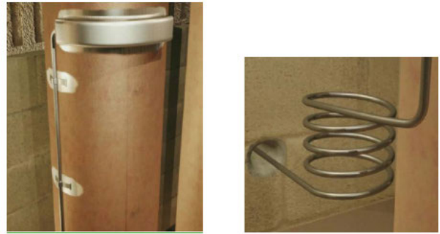
Fig. 4 : proper installation of sensor and expansion loop
